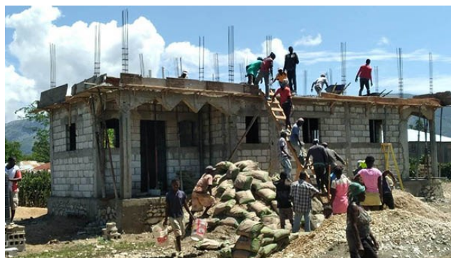
Temporary headquarters in Haiti under construction. Photo by Vildor Archange
